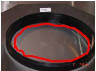
Remove the flashing, cut and remove the standing seam part of the metal roof from two inches below the lower side of the circular arc and up to the top edge of the flashing.
