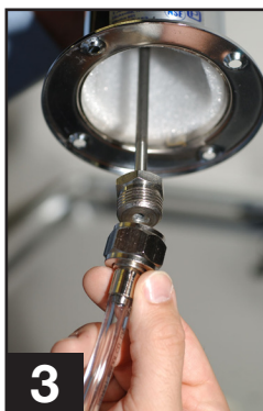
Thread beer line connector to draft arm and secure draft arm to cabinet with rubber gasket under the draft arm.
