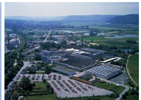
Stiebel Eltron plant in Holzminden, Germany
