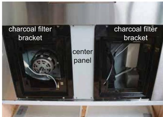
2. Using components from ZRC-0200, install (2) charcoal filter brackets and center panel to bottom of the hood with (4) screws for each component. Screws are pre-installed to the hood. Remove screws first to install brackets and center panel then re-install screws..
