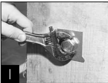
1 Removing skid from bottom of cabinet.
