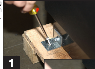
Removing bracket from cabinet.
