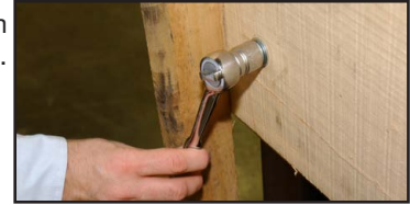
Removing skid from bottom of cabinet.
