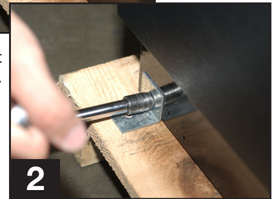
Removing bracket from cabinet.
