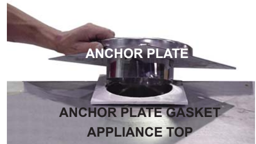
ANCHOR PLATE FOR A FACTORY BUILT CHIMNEY
