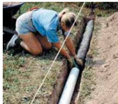
Figure 71: Underground Refrigerant Piping.
