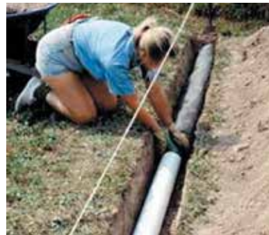
Figure 71: Underground Refrigerant Piping.
