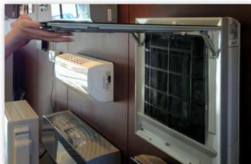
4. Lift front panel all the way. Be sure to hold with one hand at all times while removing filter.
