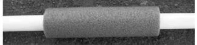
2. Place the foam pipe insulation over the fitting and crimp rings. The insulation should extend 3 inches beyond the crimp ring.
