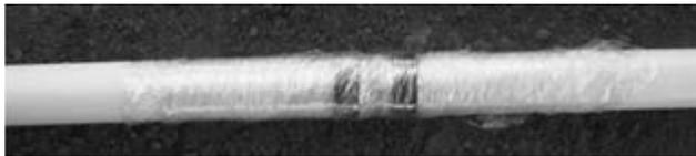
2. Wrap the fitting and crimp rings several times with the Saran wrap.
