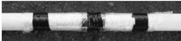
3. Tape the Saran wrap in place. Be sure the tape does not contact the ZurnPEX tubing.
