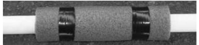
3. Tape the foam pipe insulation in place. Be sure the tape does not contact the ZurnPEX tubing.
