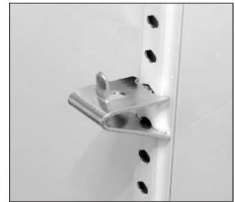
FIG. 4. Installed shelf clip.
