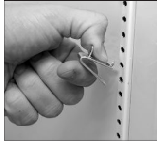
FIG. 1. Installing top tab of shelf clip.
