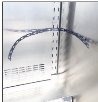
FIG. 8. Installed safety strap.
