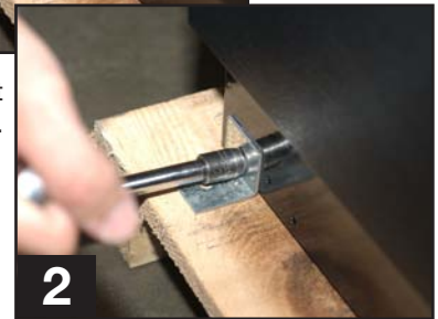
Removing bracket from cabinet.
