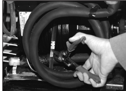
Cutting band that is around compressor
