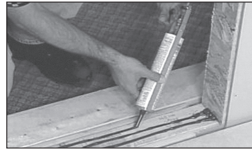
(Fig. 1-2) Caulking the sub-floor.
