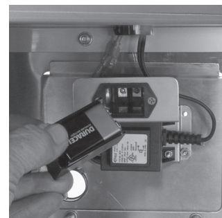
Insert and/or replace a new 9V battery
