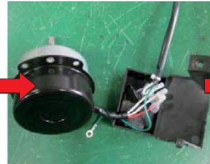
Take out the motor unit and condenser box
