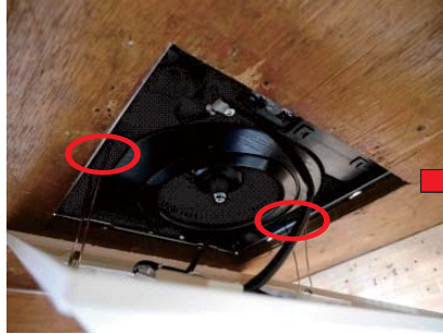
Remove the louver spring
