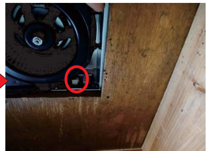
Unplug power lead connector, Then take out the casing unit from the frame assy
