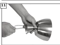
Place canopy and then yoke cover over downrod. Then thread the lead wires and safety cable from fan through the downrod as shown.
