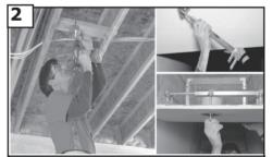
Warning-Risk of fire, electric shock, or personal injury. The fan in this box may be either directly supported from a structural framing member of a building and/or may be mounted to an outlet box marked acceptable for fan support of of 31.8kg (70 lbs) or less. Most outlet boxes commonly used for the support of lumminaires may not be acceptable for fan support and may need to be replaced. Consult a qualified electrician if in doubt.
