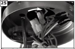
Install the switch housing cover by aligning the 2 screws with the 2 key slot holes on the plate and twist to lock into place. Install the 1 screw removed and tighten the other 2 screws securely.
