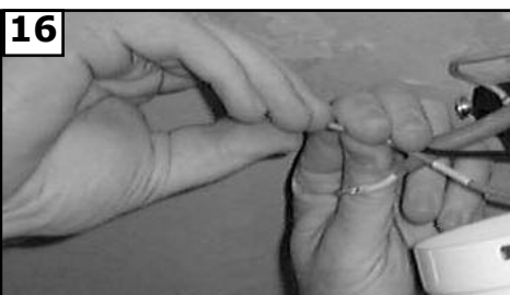
Make wire connections to power source using wire nuts provided. Make sure that no filaments are outside of the wirenut. After making the wire connections, the wires should be spread apart with the grounded conductor and the equipment-grounding conductor on one side of the outlet box and ungrounded conductor on the other side of the outlet box. The splices after being made should be turned upward and pushed carefully up into the outlet box.
