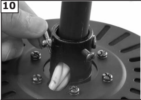
10 Install keeper pin.
