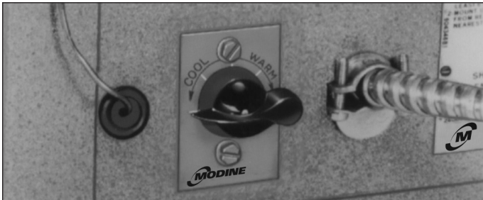
Figure 9.1 - Unit-Mounted Thermostat
