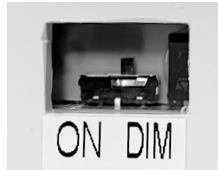
Left side of wall control
