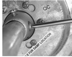
reinstall stopper screw and tighten set screw
