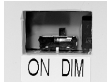
Left side of wall control
