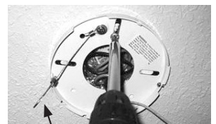
suspension cable and loop
