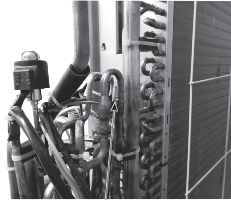
Thermistor <Outdoor liquid pipe> (TH3)
