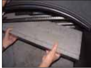
Tilt Baffle downward towards front of fireplace
