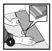
After thoroughly cleaning the subfloor, you should begin laying from left to right. Position the first plank so that grooved edge is facing you.
