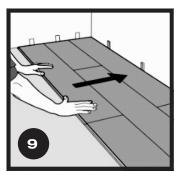
After the first 2-3 rows of planks are installed, they should be checked with a string line to ensure that rows are still running straight. If they are not, it could be that the starting wall has some irregularities that caused bowing in the installation.
