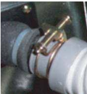
Clamp the Flexible Drain Hose Connection
