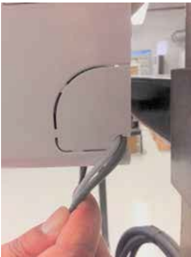
Figure 90: Indoor Unit Knockout (Communication Wires)
