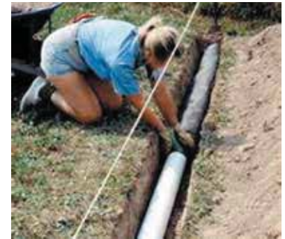
Figure 65: Underground Refrigerant Piping.
