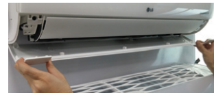
Figure 98: Checking that All Attachment Locations Are Secure (Step 5).
