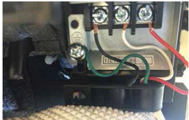
Figure 91: Indoor Unit Terminal Block with Grounding Cable (Example Only)
