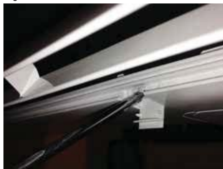
Figure 89: Remove (and Reattachment) Bottom Panel
