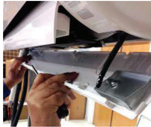
Figure 16: Remove Bottom Panel.
