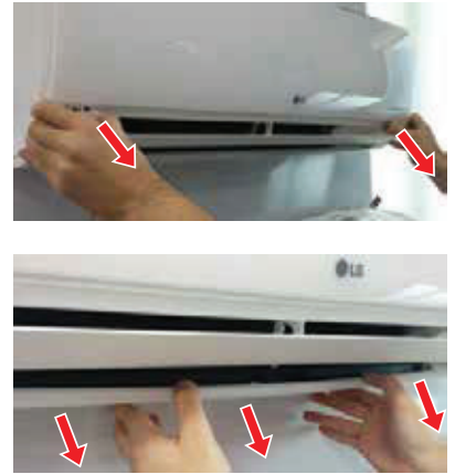
Figure 18: Removing the HSV5 Bottom Cover (Appearances Will Vary Depending on Indoor Unit Model).
