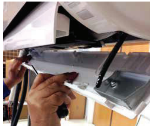
Figure 16: Remove Bottom Panel.
