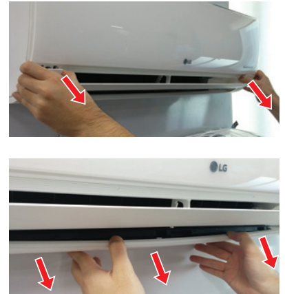
Figure 17: Removing the Bottom Cover (Appearances Will Vary Depending on Indoor Unit Model).
