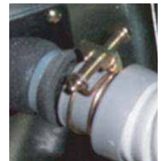
Clamp the Flexible Drain Hose Connection
