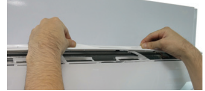
Figure 99: Disassembling the Air Filter (Appearances Will Vary Depending on Indoor Unit Model).
