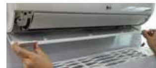
Figure 96: Checking that All Attachment Locations Are Secure (Step 5).
