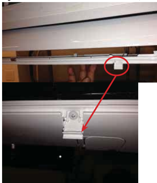
Figure 88: Remove Screws from Bottom Panel
