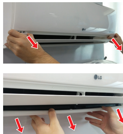
Figure 17: Removing the Bottom Cover (Appearances Will Vary Depending on Indoor Unit Model).
