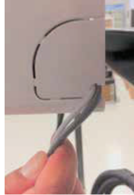
Figure 74: Indoor Unit Knockout.
