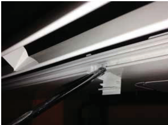
Figure 72: Remove Screws from Bottom Panel.
