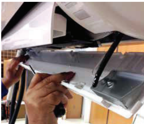
Figure 73: Remove Bottom Panel.
