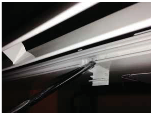
Figure 15: Remove Screws from Bottom Panel.
