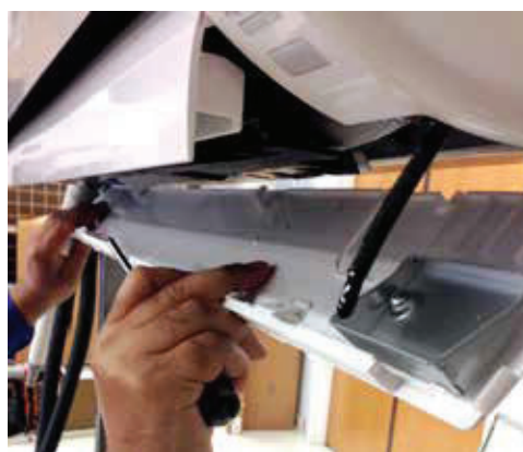
Figure 16: Remove Bottom Panel.
