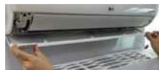
Figure 96: Checking that All Attachment Locations Are Secure (Step 5).
