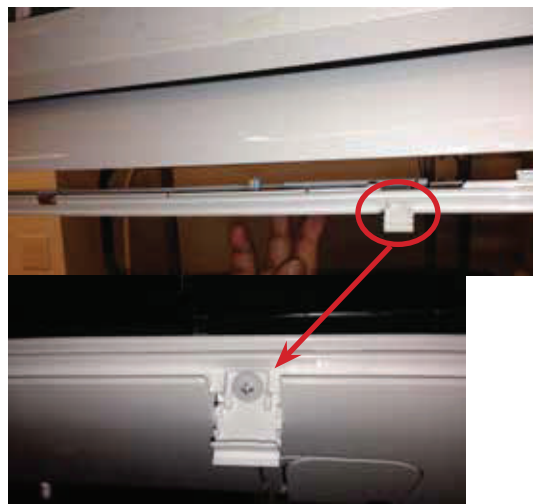
Figure 14: Latch over Screws on Indoor Unit Bottom Panel.
