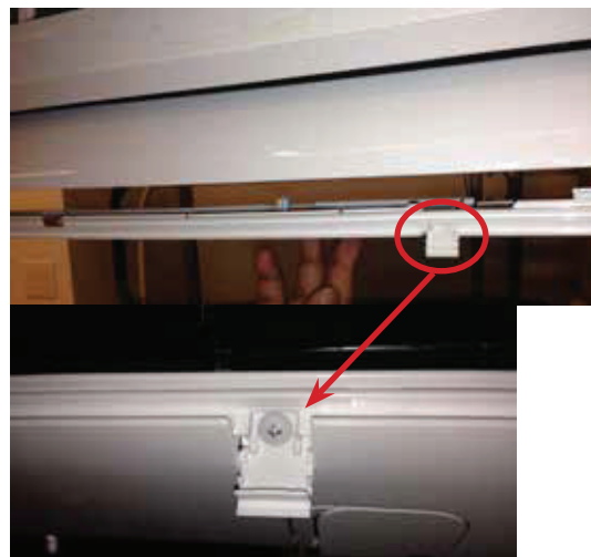
Figure 71: Latch over Screws on Indoor Unit Bottom Panel.
