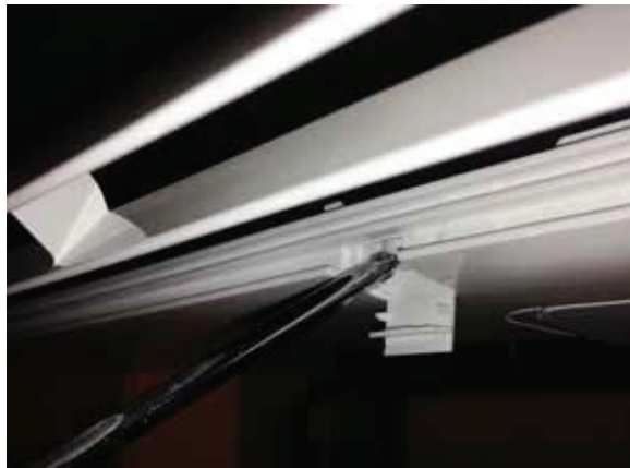
Figure 72: Remove Screws from Bottom Panel.
