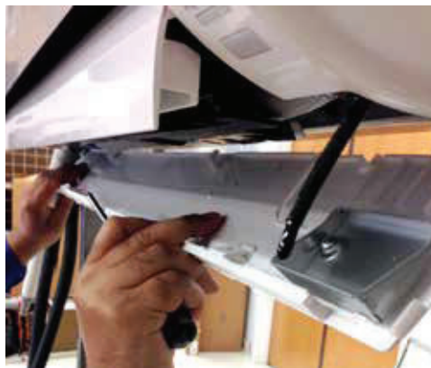
Figure 73: Remove Bottom Panel.
