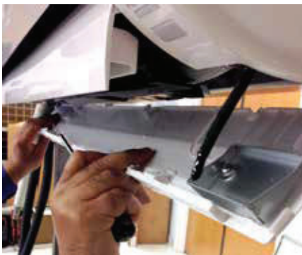
Figure 89: Reattaching the Bottom Panel.
