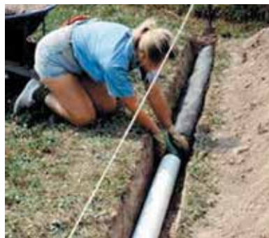
Figure 38: Underground Refrigerant Piping.
