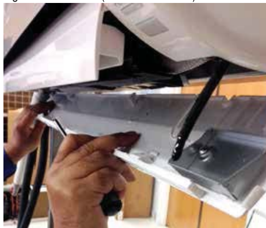
Figure 89: Remove (and Reattachment) Bottom Panel
