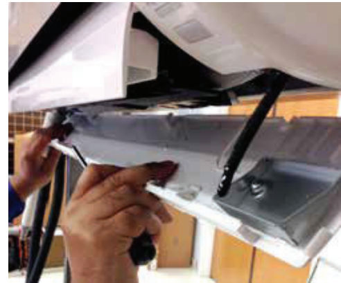
Figure 16: Remove Bottom Panel.
