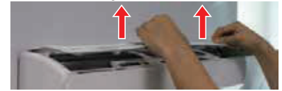
Figure 98: Assembling the Air Filter (Appearances Will Vary Depending on Indoor Unit Model).
