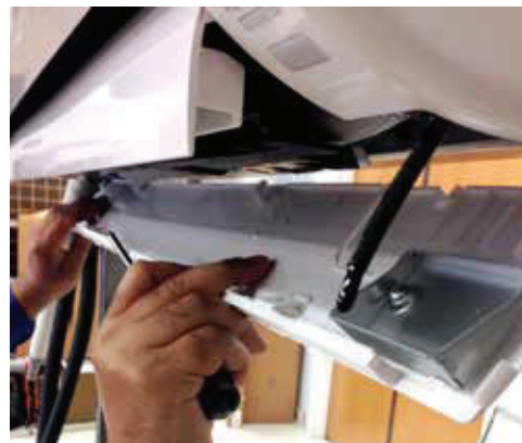
Figure 73: Remove Bottom Panel.
