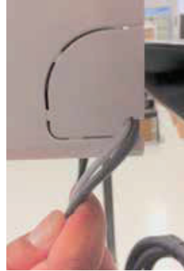
Figure 74: Indoor Unit Knockout.
