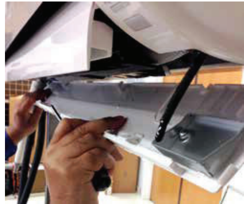
Figure 16: Remove Bottom Panel.
