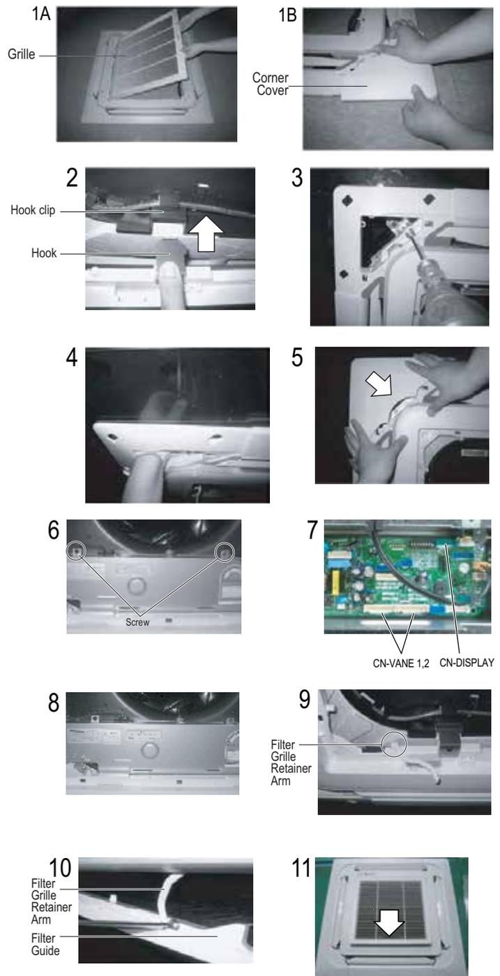
Figure 58: Ensure that no gaps are present between the indoor unit frame and the decoration grille.
