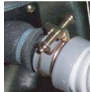
Clamp the Flexible Drain Hose Connection
