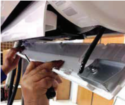
Figure 89: Reattaching the Bottom Panel.
