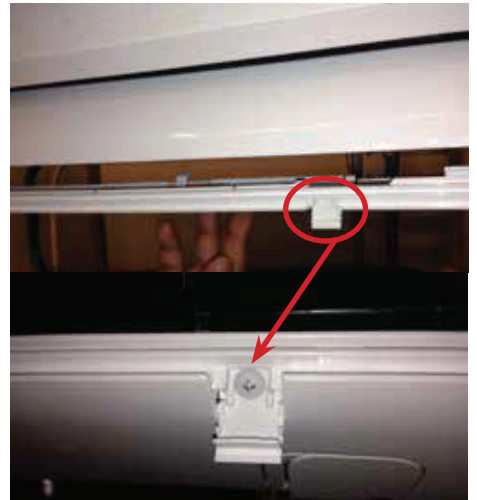
Figure 91: Reattaching the Screws on the Bottom Panel.
