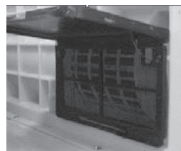
Figure B – Vent Filter Removal
