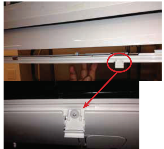
Figure 71: Latch over Screws on Indoor Unit Bottom Panel.
