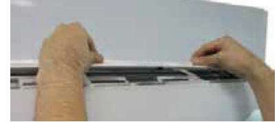
Figure 97: Disassembling the Air Filter (Appearances Will Vary Depending on Indoor Unit Model).
