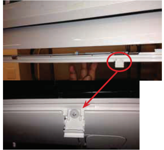
Figure 14: Latch over Screws on Indoor Unit Bottom Panel.
