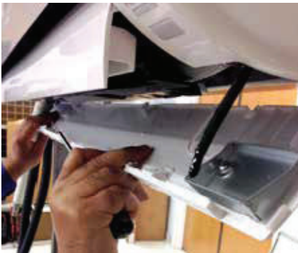
Figure 89: Reattaching the Bottom Panel.
