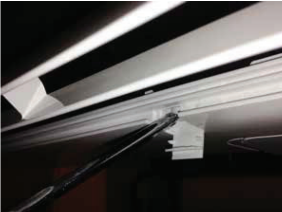
Figure 15: Remove Screws from Bottom Panel.
