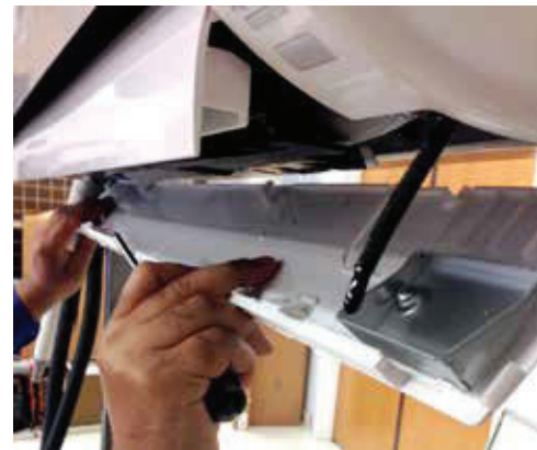
Figure 16: Remove Bottom Panel.
